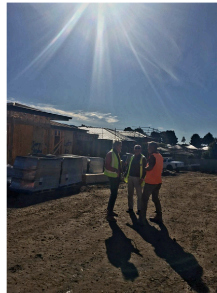
Geoff Reeve on site with incoming residents
